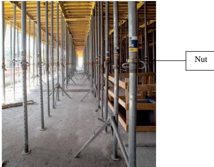
Figure 6: Adjustable props
