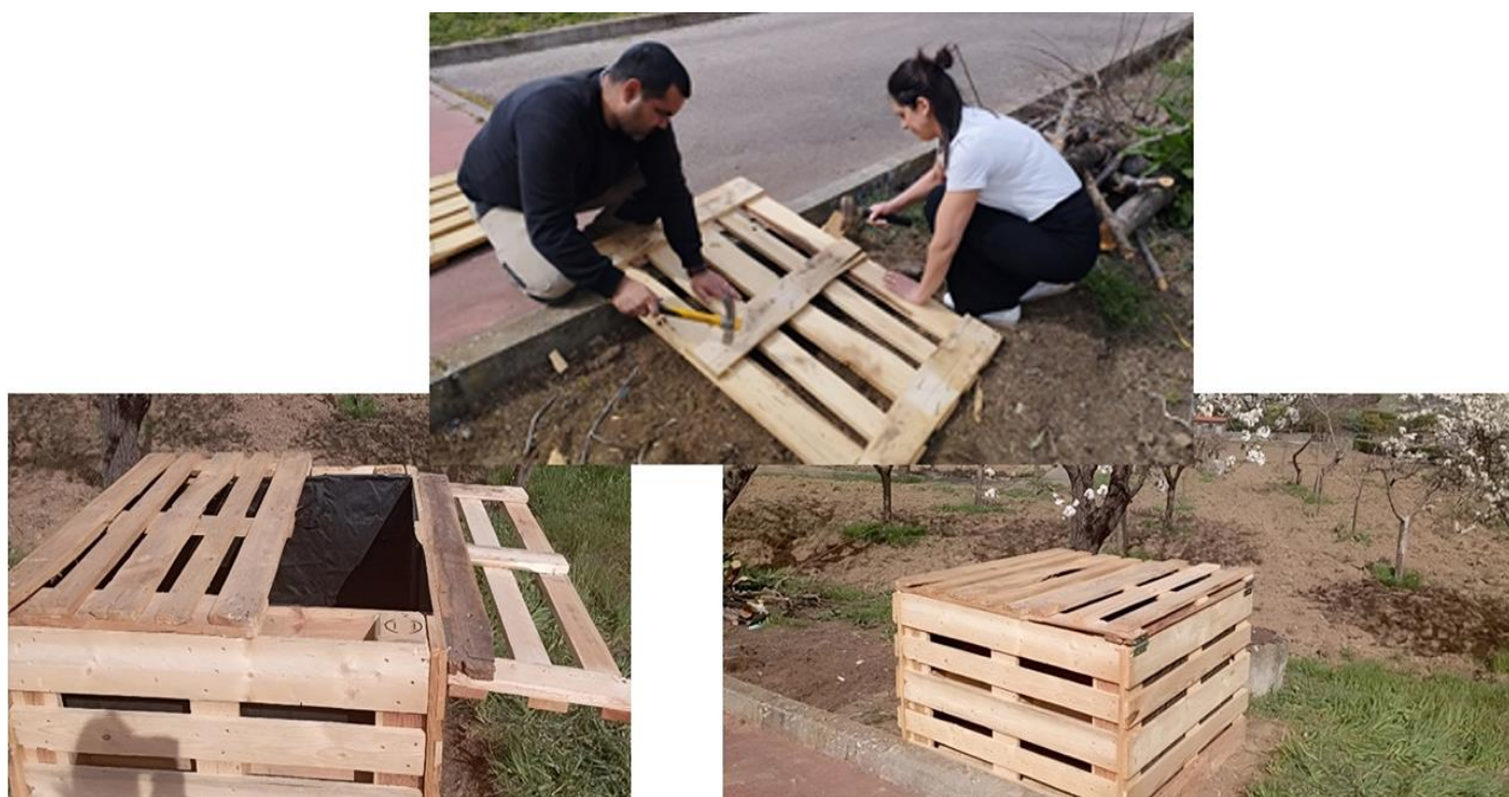
Figure 3. Construction & final result of composter (photograph taken by the authors)
