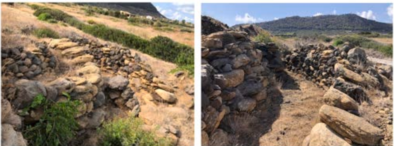
Fig. 7. Left) Outer and right) inner structure of Tower No. 12.
