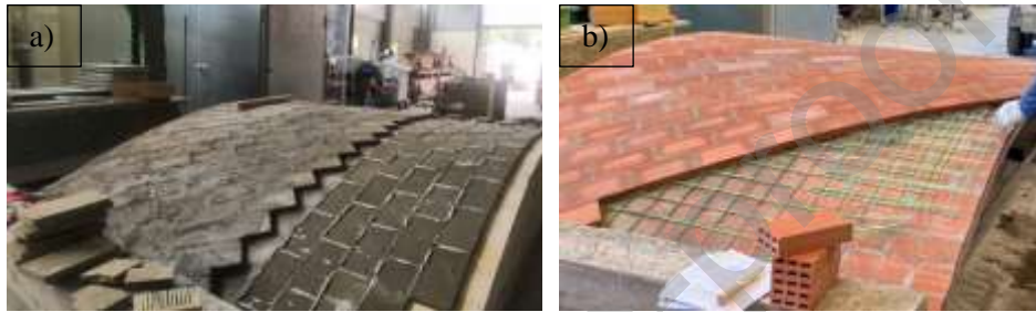
Fig. 10. Vault fabrication: a) V-ER, b) V-RM.
