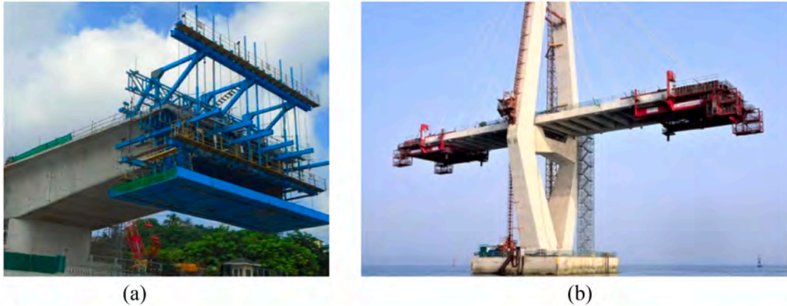
Fig. 4. a: Overhead formwork traveller (OH) b: Underslung formwork traveller (US).
