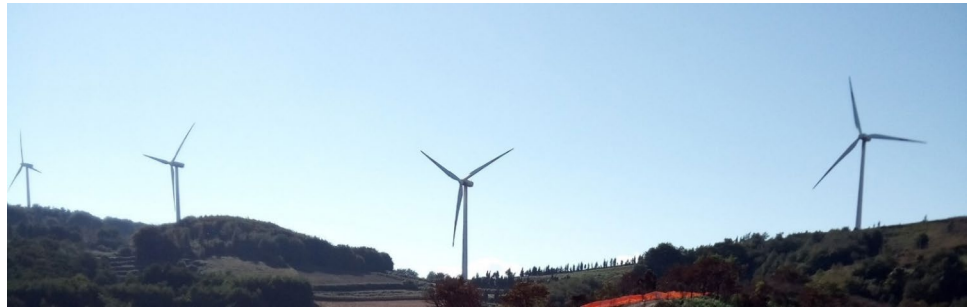
Fig. 1 Example of a wind farm ( www.sevasrl.it )
