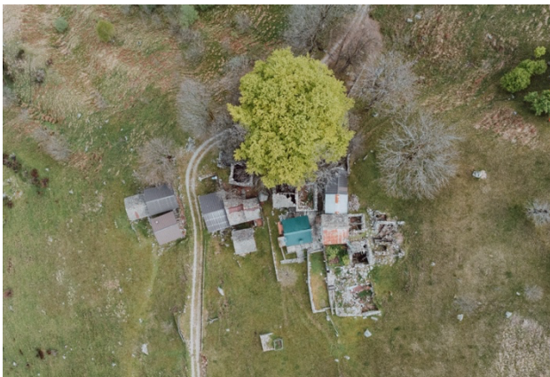
Figure 2. The marginalization process in the Inner Areas leads to the loss of heritage, as happens with these rural buildings in the Italian Alps (image L. Pozzoni 2023).
