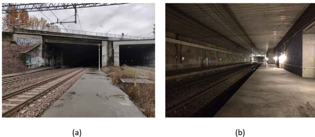
Fig. 1. Overview of railway tunnel: north entrance (a) and internal geometry near the platform (b).
