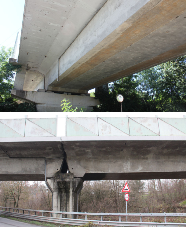
Figure 1: PC box-girder railway bridge.
