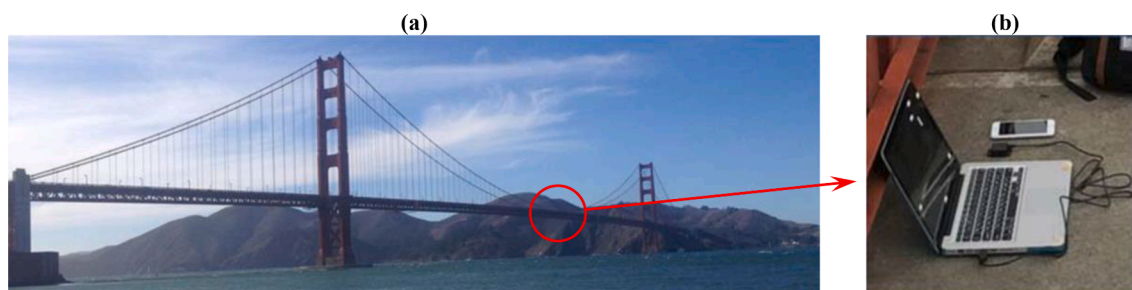
Fig. 8. Smartphone-based modal identification by Ozer et al. [78]: (a) the monitored structure (i.e., the Golden Gate Bridge), (b) the devices of the fixed contact-based measurement technique.
