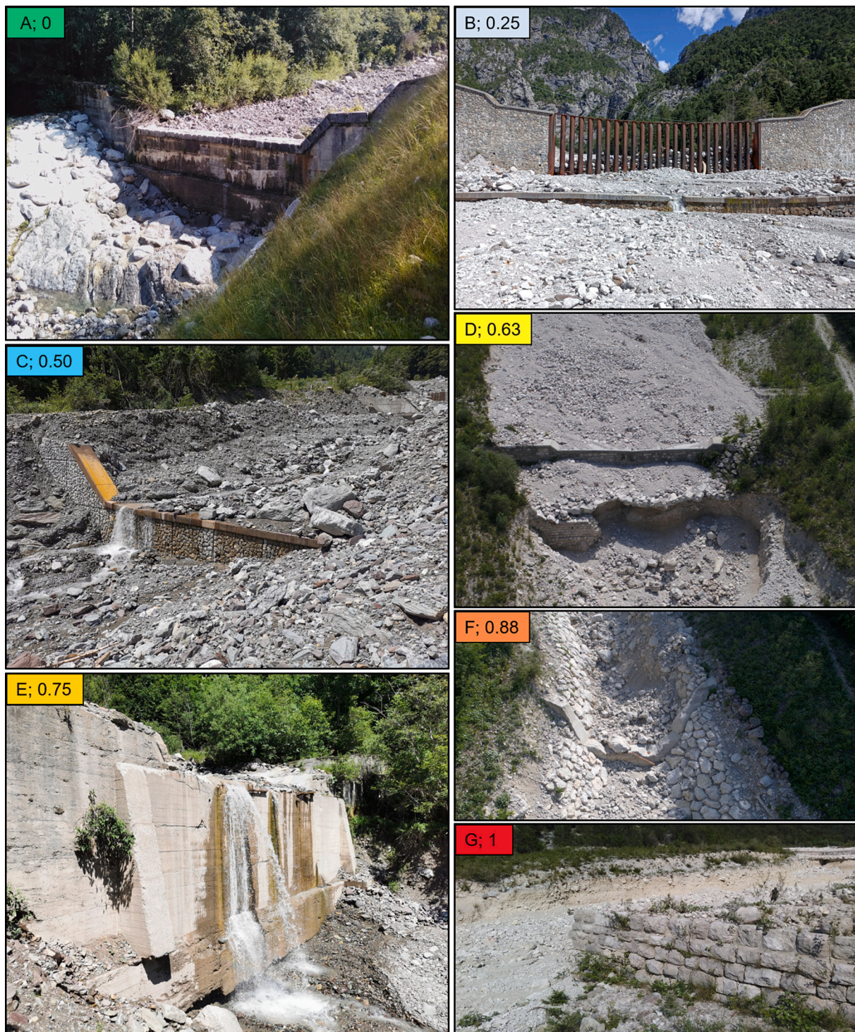
Fig. 6. Examples of check dams with different MPI values associated. (A) Check dam A120 in the Agozza Torrent was assigned 0 of the MPI and green-rank. (B) Open check dam U060 in the Uccelli Torrent was assigned 0.25 of the MPI and blue-rank. (C) Check dam M130S in the Miozza Torrent was assigned 0.5 of the MPI and blue-rank. (D) Check dam V060 in the Vegliato Torrent was assigned 0.63 of the MPI and orange-rank. (E) Check dam M100S in the Miozza Torrent was assigned 0.75 of the MPI and red orange-rank. (F) Bed sill V190 in the Vegliato Torrent was assigned 0.88 of the MPI and orange-rank. (G) Check dam V050 in the Vegliato Torrent was assigned 1 of the MPI and red-rank. Photos taken in summer 2022. (For interpretation of the references to colour in this figure legend, the reader is referred to the web version of this article.)
