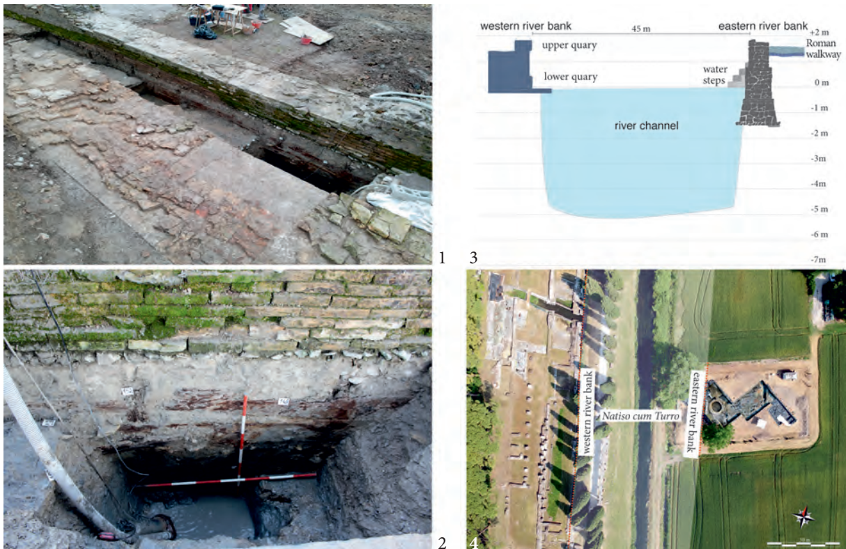
Fig. 5: Aquileia river port. 1 – The Republican city walls on the left and the western wall of the storehouse on the right (photo Archeotest). 2 – The formwork and the foundations of the western wall of the storehouse (photo Archeotest); 3 – Simplified section of the monumental fluvial channel with its eastern and western banks (by A. Cipolato); 4 – River port in Aquileia, an overview of the area with indication of the width of the palaeo-riverbed (from Cottica, Cipolato 2023).
