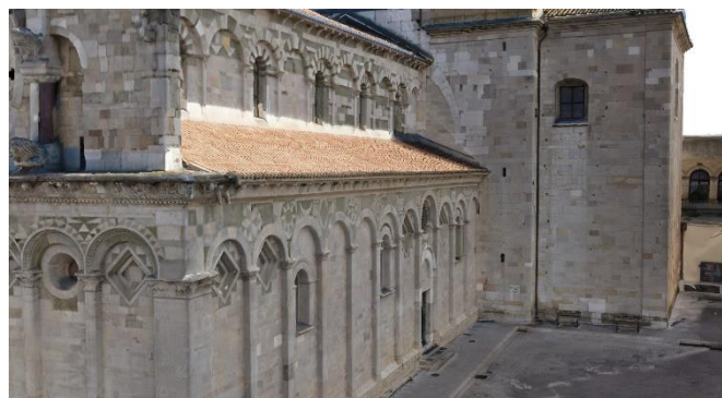
Figure 6. Textured 3D model obtained by terrestrial and aerial drone photogrammetry.
