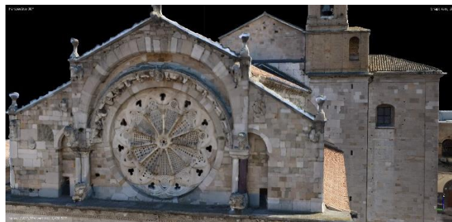
Figure 5. Drone acquisition: textured model, zoom of the rose window of the main elevation on Regina Margherita Street.
