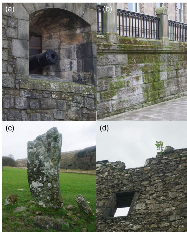
FIGURE 5 Pollution soiling and biological colonization on stone; at Edinburgh Castle, Scotland, UK (a) © Photo by Dr. Elena Sesana; on Elmbank street, Glasgow, Scotland, UK (b) © Photo by Dr. John Hughes; at Large standing stones (c) © Photo by Dr. Elena Sesana; and at Kilchurn Castle, Scotland, UK (d) © Photo by Dr. Elena Sesana
