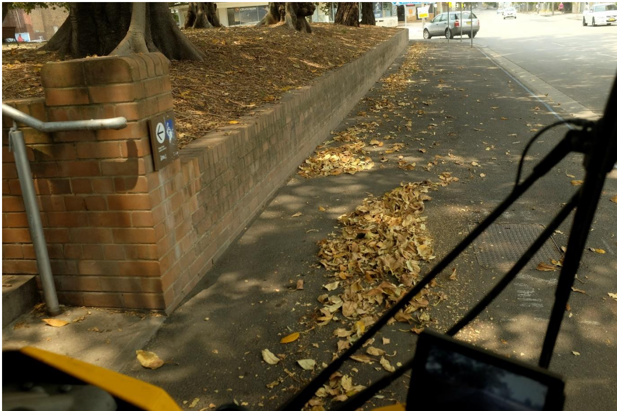
Photograph 41: Bridge Road in Ultimo, footpath under the Moreton Bay Fig Trees
