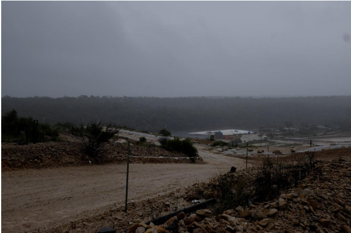
Photograph 73: The leachate dam at the bottom of the hill
