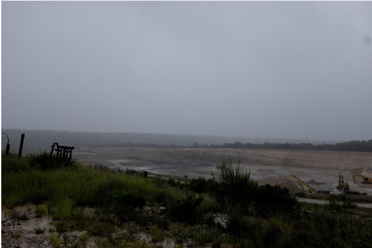
Photograph 74: A 'to-be-filled' section of the landfill
