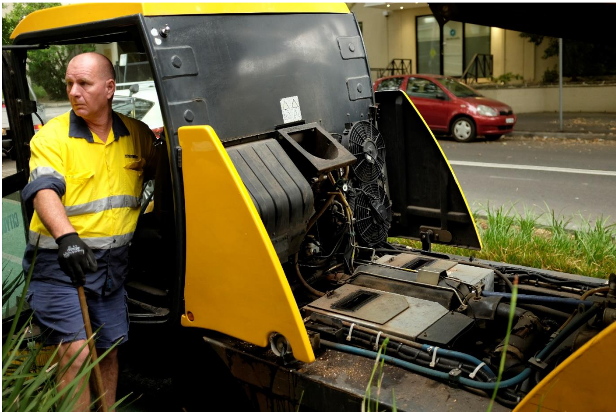
Photograph 33: Opening the Footway
