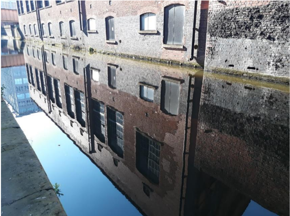
Figure 29: Bloom Street Power Station
