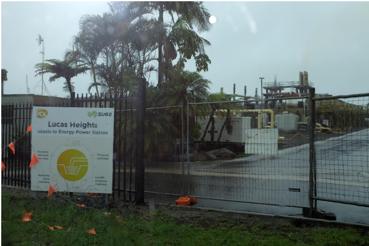
Photograph 79: Lucas Heights Waste to Energy Power Station, at the at the Lucas Heights Resource Recovery Park
