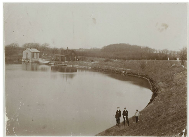
Fig. 2 The Oranjekom (Orange bowl; photographed in 1909), which was excavated by the Dunewater Company and named after King Willem van Oranje, who (as the 11-years-old crown prince) dug the first sod in the ground at the construction site of the first centralised drinking water production facility in the Netherlands (obtained from Noord-Hollands Archief, 1100 – Image collection of the municipality of Haarlem, inventory number 38723)
