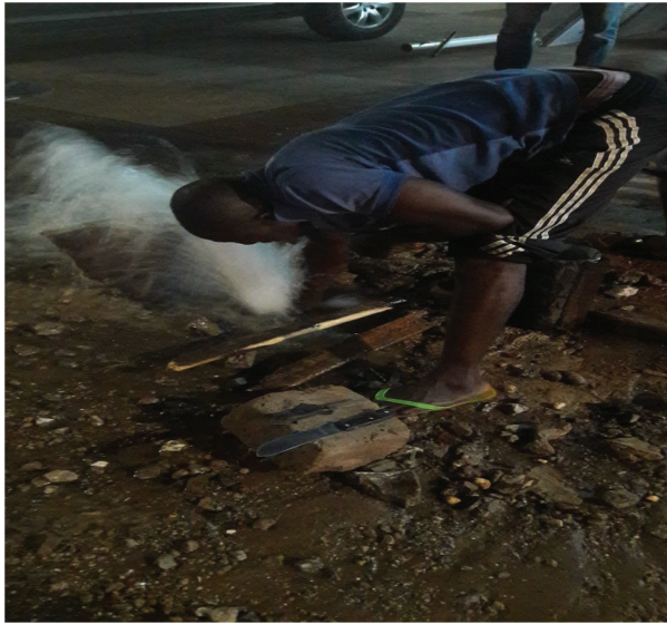
Figure 6. Private plumber repairing a burst pipeline in Nima (March 10, 2020).
