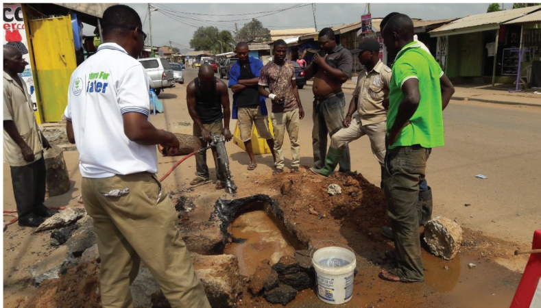
Figure 4. GWCL’s officials repairing a pipeline, Accra–Agbogba junction (December 8, 2018).
