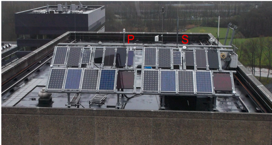
Fig. 6. Experimental setup at Utrecht University, Utrecht, the Netherlands. P denotes locations of pyranometers, S of the spectroradiometer.
