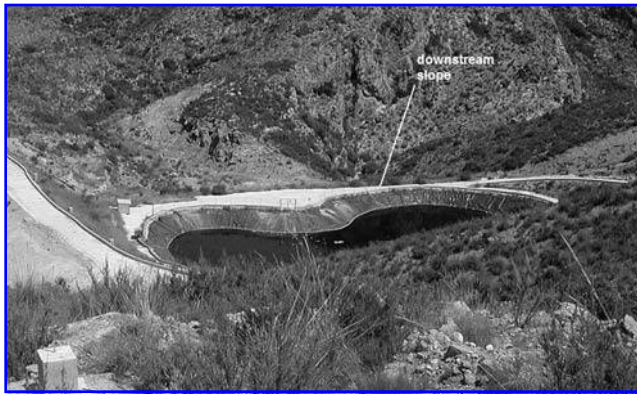
FIG. 9. Leachate dam for a rejects landfill.
