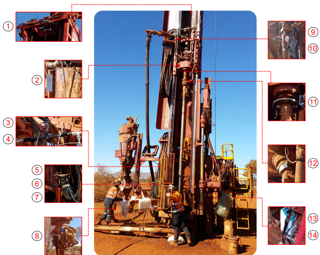
Figure 3.4: Schramm rotary drilling rig T685WS and location of sensors.
