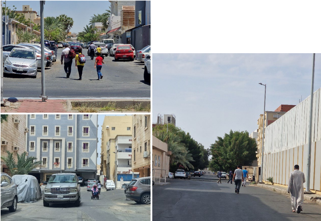
Figure 6-40. Pedestrians have no choice but to walk along with automobiles due to the absence or inadequacy of sidewalks.
