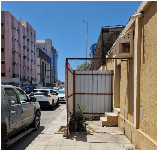
Figure 6-28. A partition that provides privacy for a school guard's room while also encroaching on the sidewalk zone.
