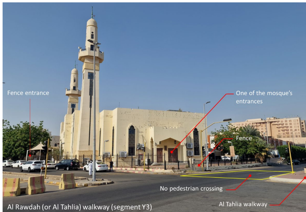
Figure 6-61. Prioritisation of pedestrians' accessibility would be via fence removal, creating a pedestrian crossing, and reducing traffic speed.
