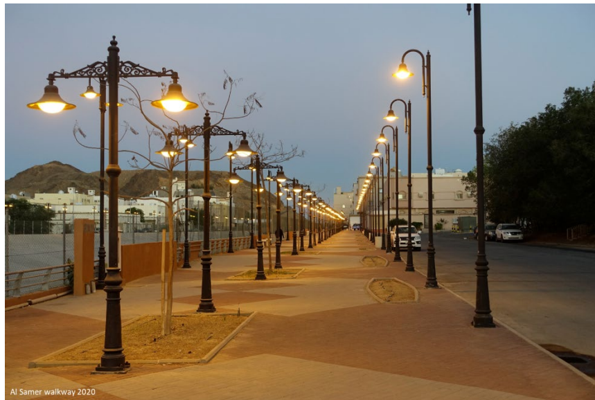
Figure 6-12. Another example of the road-like provision of lighting fixtures.
