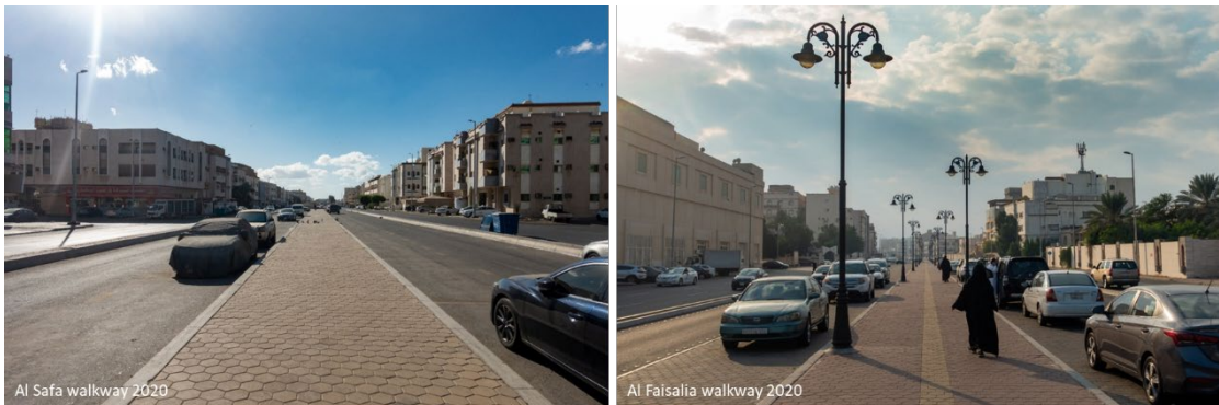
Figure 6-9. With two driveways (each direction) and parallel parking bays, the space dedicated to pedestrians is approximately one-fifth of the total width.
