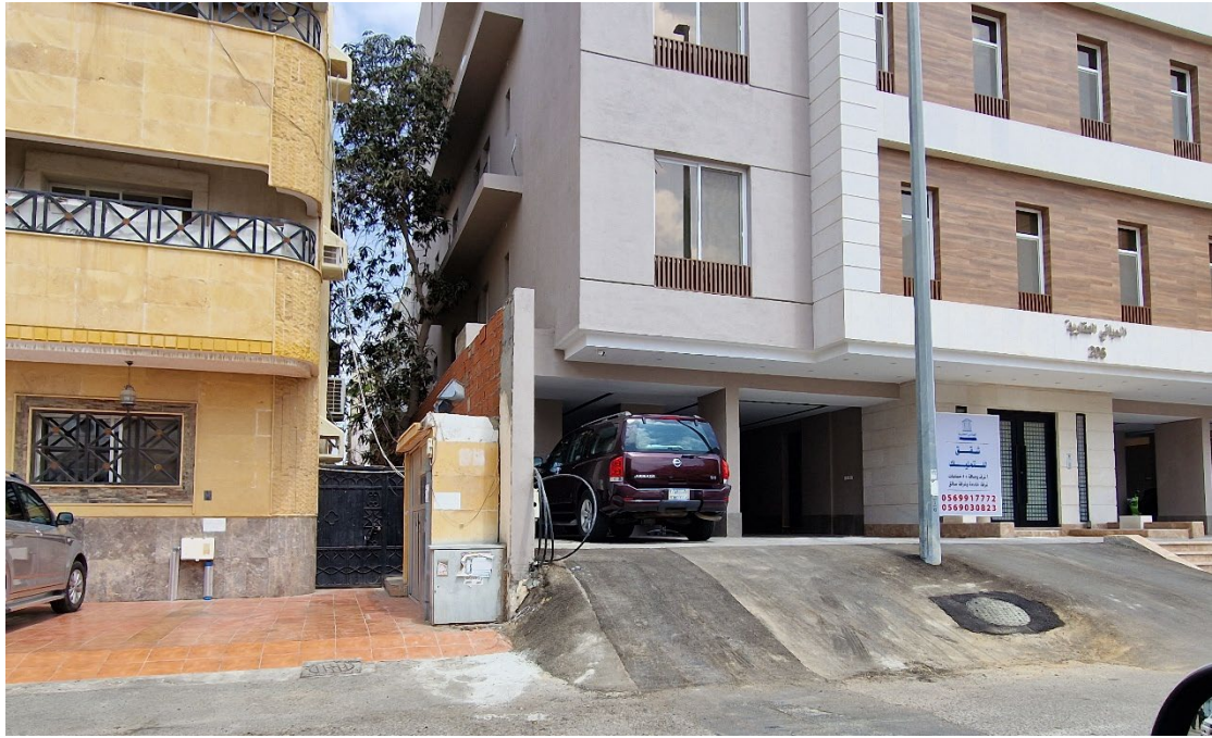
Figure 6-42. The regulation that permitted creating vehicle parking at the ground floor level of residential buildings did not consider its compatibility with the buildings' setback requirements and relationship to streets.
