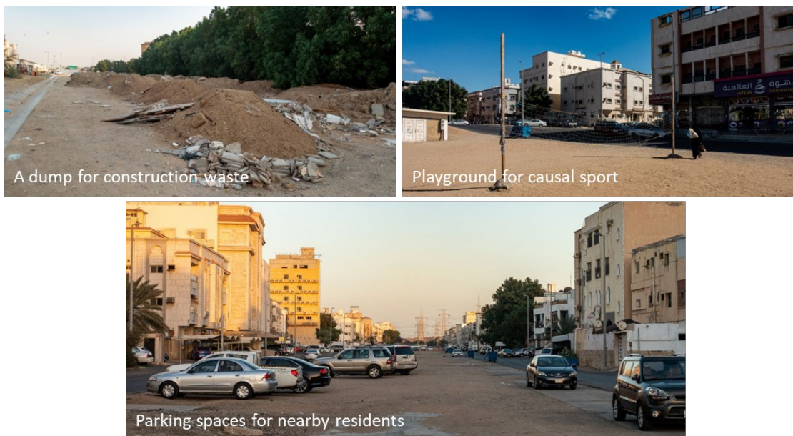
Figure 6-6. Examples of how undeveloped (or idle) segments of the Northern Drainage Channel are used (Jan 2020).
