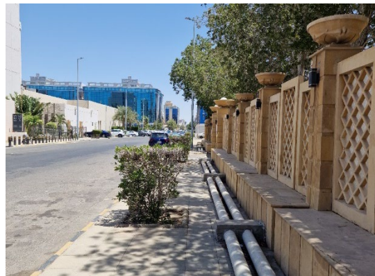
Figure 6-35. The placement of pipes and planters reduce sidewalk's effective pedestrian zone to less than 0.7 m.
