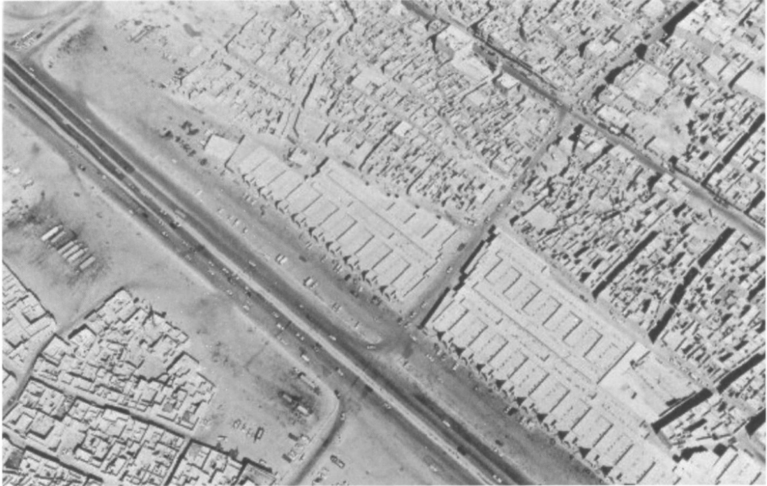
Figure 3-8. Spatial qualities that defined Riyadh's traditional Arab-Muslim urban fabric during the 1960s were disrupted via wide roads and large malls (Al-Hemaidi, 2001).
