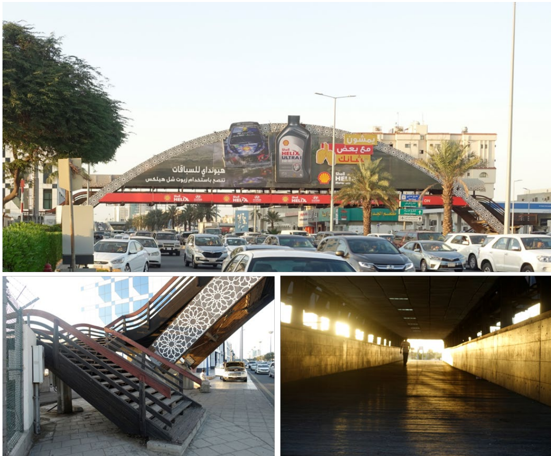
Figure 9-1. Pedestrian bridge on Al Madian Road, near Al Rawdah walkway.
