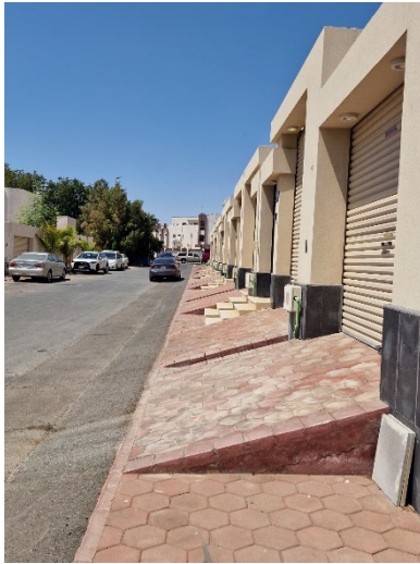
Figure 6-25. Stairs and driveways of single-family dwellings in Al Rawdah neighbourhood make the presented sidewalk un-walkable.
