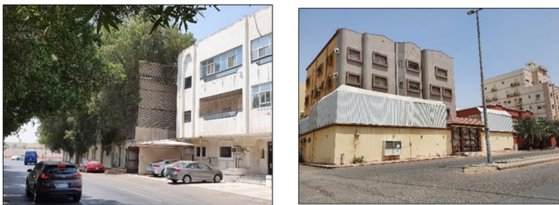
Figure 2-7. examples of walled residential units in Jeddah city (Shawly, 2022).
