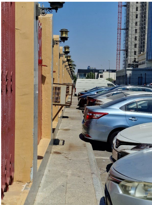
Figure 6-30. Sidewalk obstructions caused by air conditioning units and parked cars.
