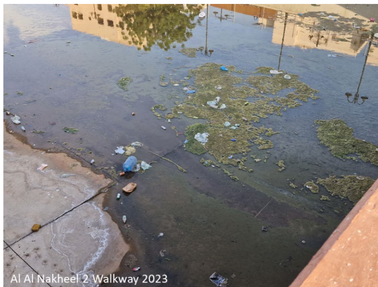
Figure 7-22. Nearly stagnant, untreated, and unfiltered water can indirectly harm walkway/LP users (or nearby residents) by becoming a breeding ground for mosquitos that can transmit diseases.
