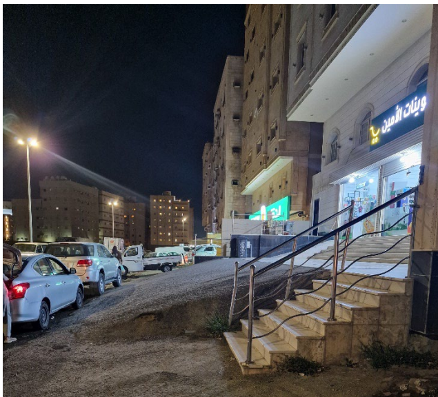
Figure 6-41. The elevation difference between buildings' ground floor and streets hinders pedestrians' movement—vehicle ramps, like in the exhibited case, encroach streets' right-of-way.
