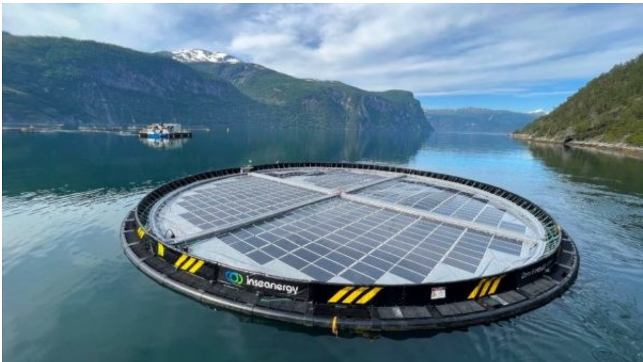
Figure 1.10: FSPV System Installed in Norway for Aquaculture Site
