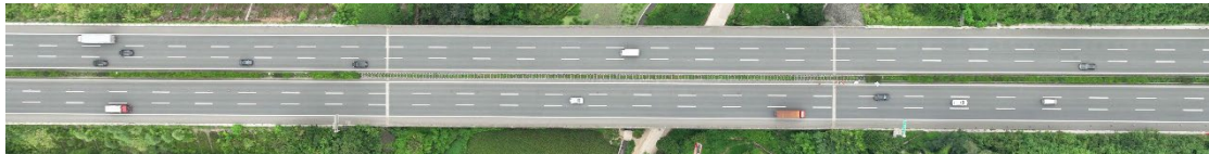
Fig. 16. Top view of location 3
