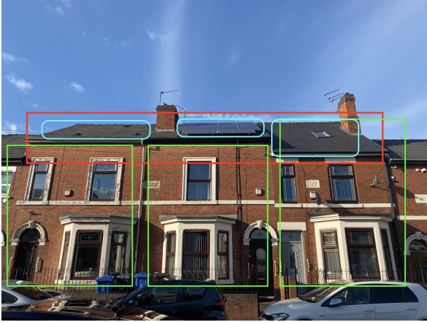
Fig. 3: A example of terraced houses seperation problem
