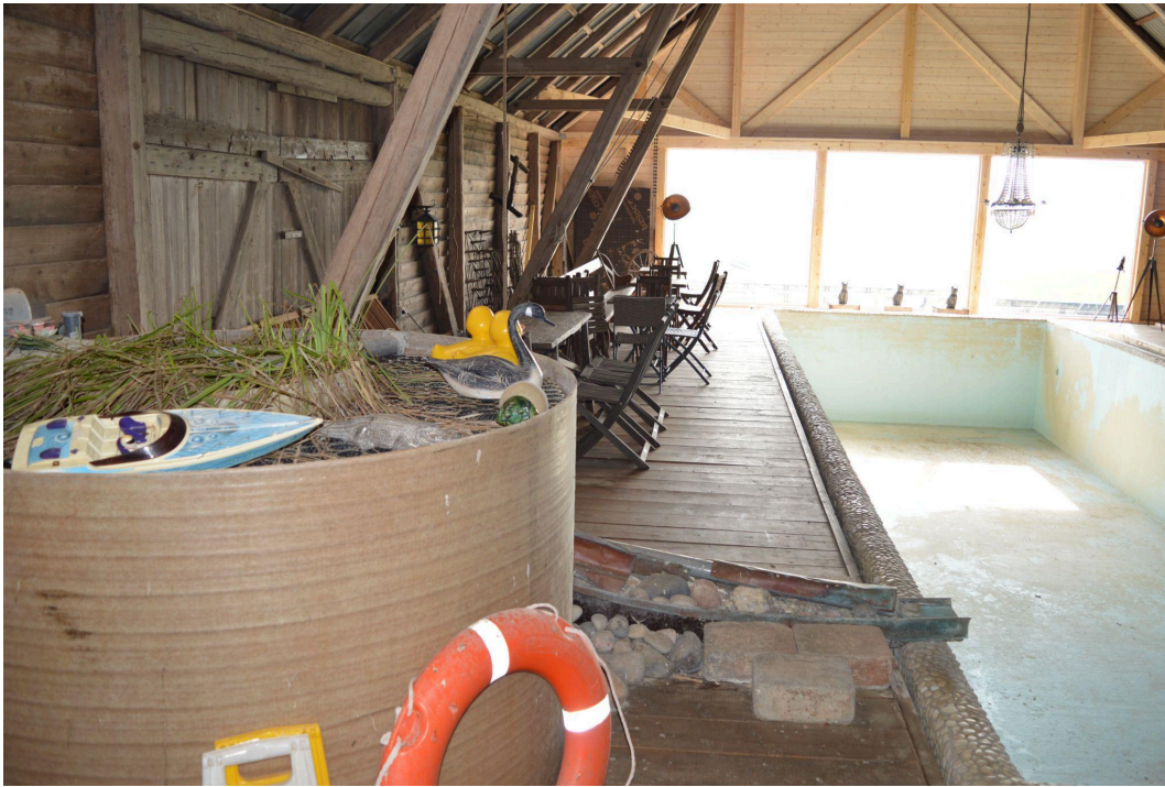
Figure 3. Hybrid filter system (left of the picture) which is connected to rainwater. (The picture was taken by: Ernő Tóth-Pál)
