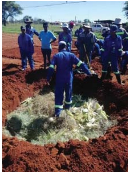
Figure 3.19. Preparing a large trench bed on the TAC campus, using waste from maize harvesting as an organic material layer
