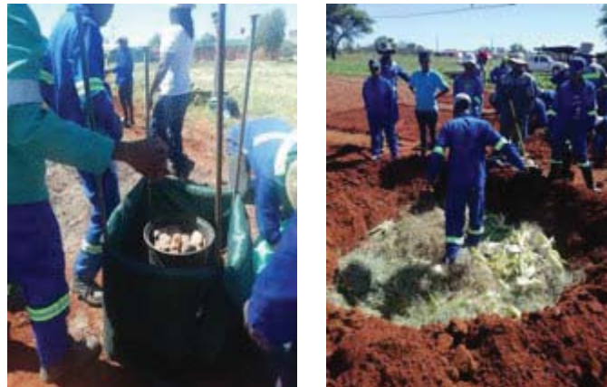
Figure 4.39. Tower garden and trench bed construction at TAC
