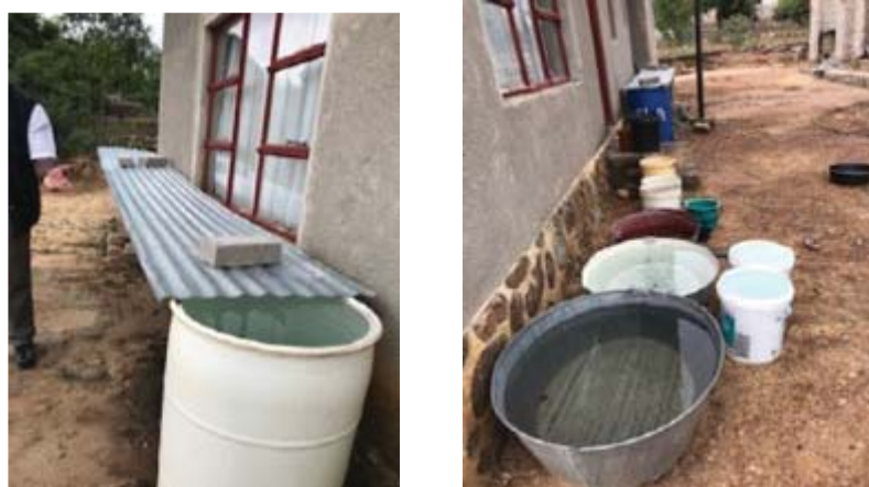
Figure 3.11. Typical strategies for collecting rainwater for use in households and gardens observed in Mpumalanga former homeland areas
