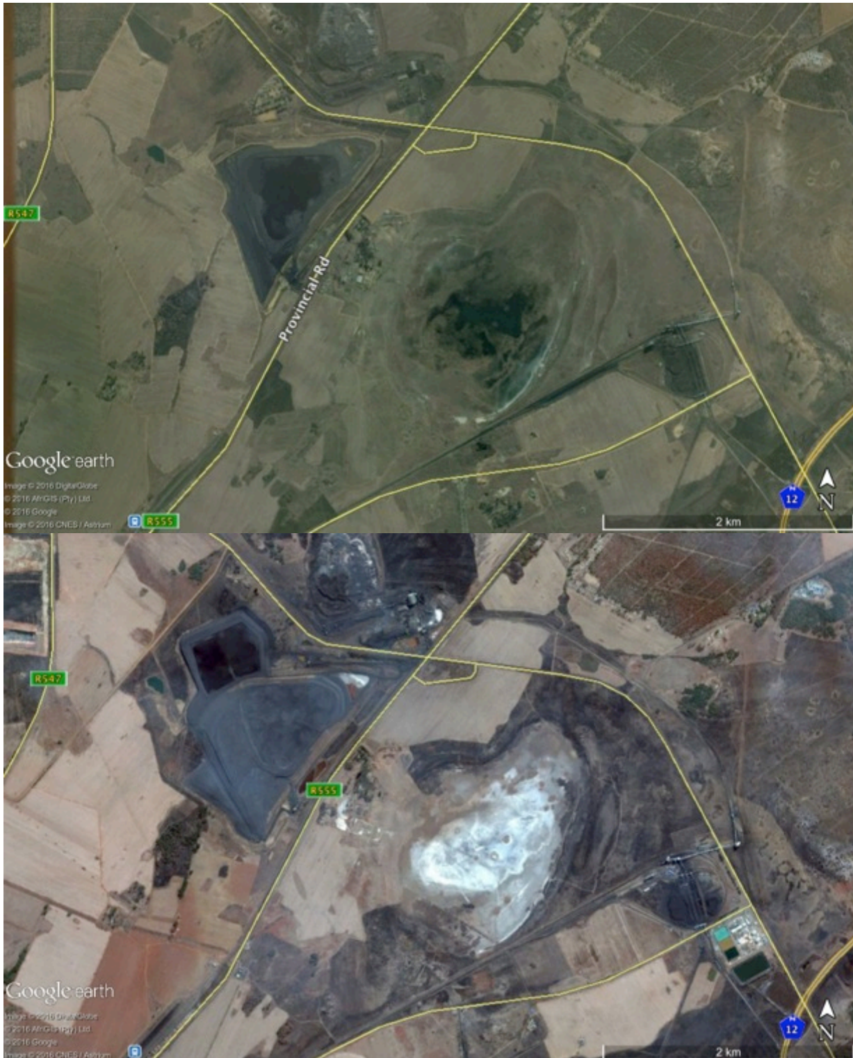
Figure 62 Pan system before mine water impact (top) and after disposal of sulphate rich mine water (bottom)
