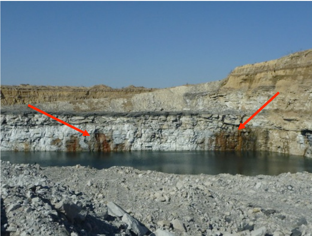
Figure 20 Opencast mine profile indicating a distinct flow path (arrows) in the bedrock
