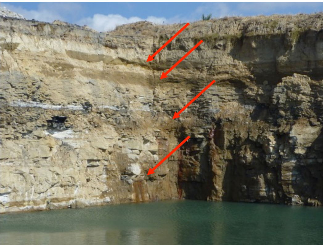
Figure 21 Opencast mine profile indicating numerous distinct flow paths (arrows) through the exposed profile (soil, weathered sandstone, carbonaceous shale, hard sandstone)
