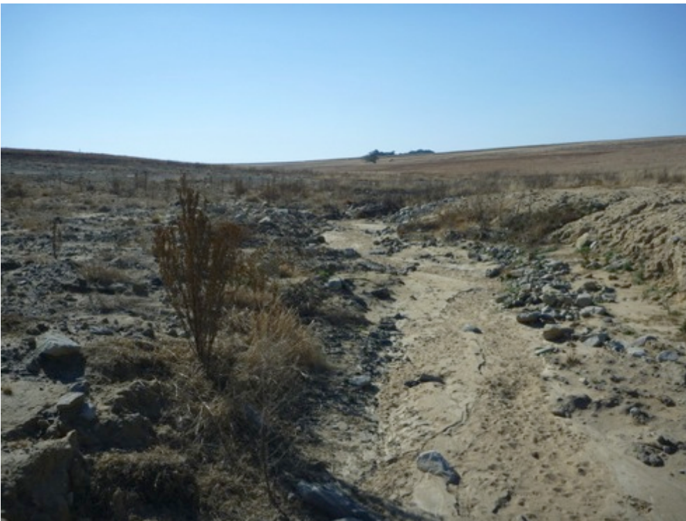
Figure 41 Eroded channel (gully erosion) of the unnamed tributary of the Holbankspruit on the in-filled wetland site
