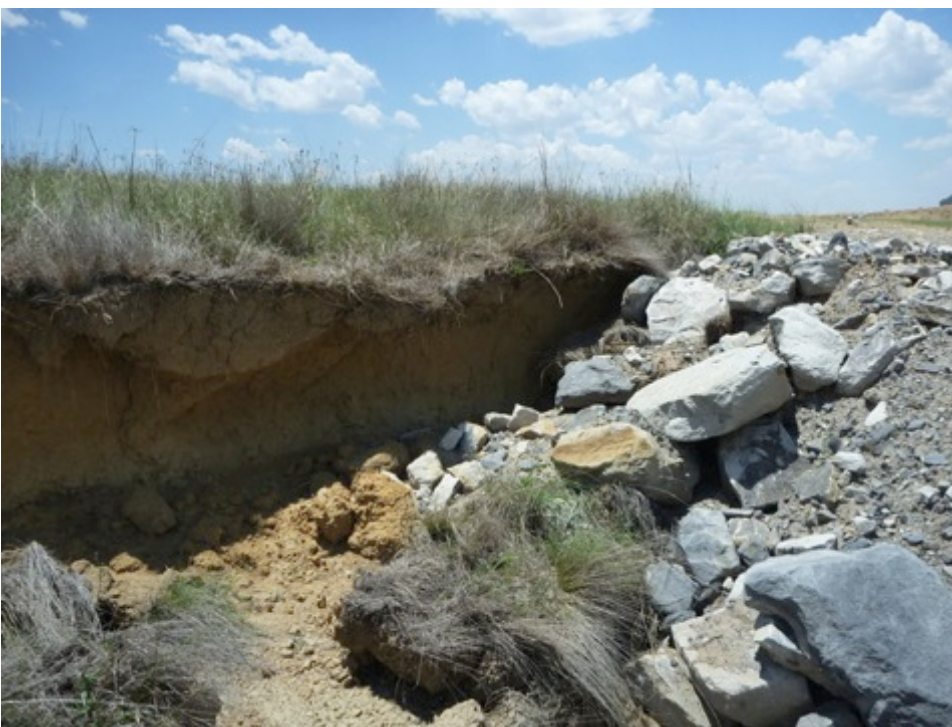
Figure 35 Wetland area filled-in with mine spoil material
