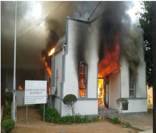
Figure 1-11: The offices of the Sundays River Valley Municipality in Kirkwood, Eastern Cape, were destroyed by arson as part of public water protests. Photo 23/09/2014. Source: Facebook (no citation/acknowledgement available). (Clifford-Holmes et al., 2015).
