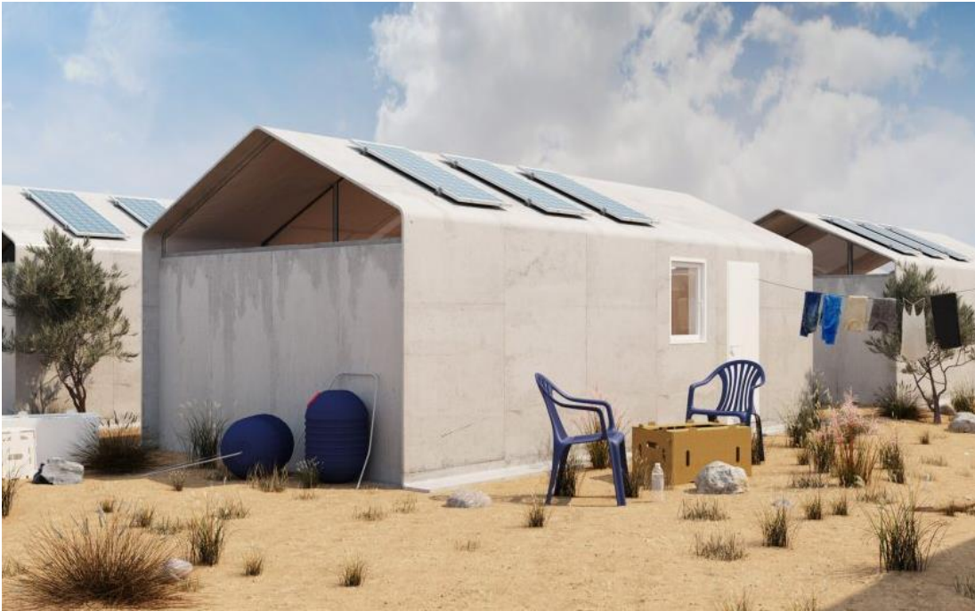
Figure 58: Exterior of One Living Pod
