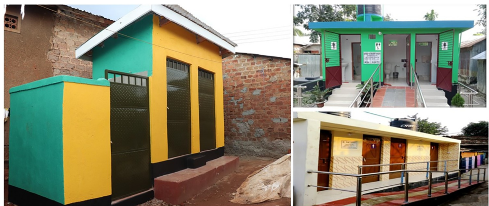
Fig 1. Shared sanitation facilities implemented across informal settlements in Bangladesh, Kampala, and Nairobi.
