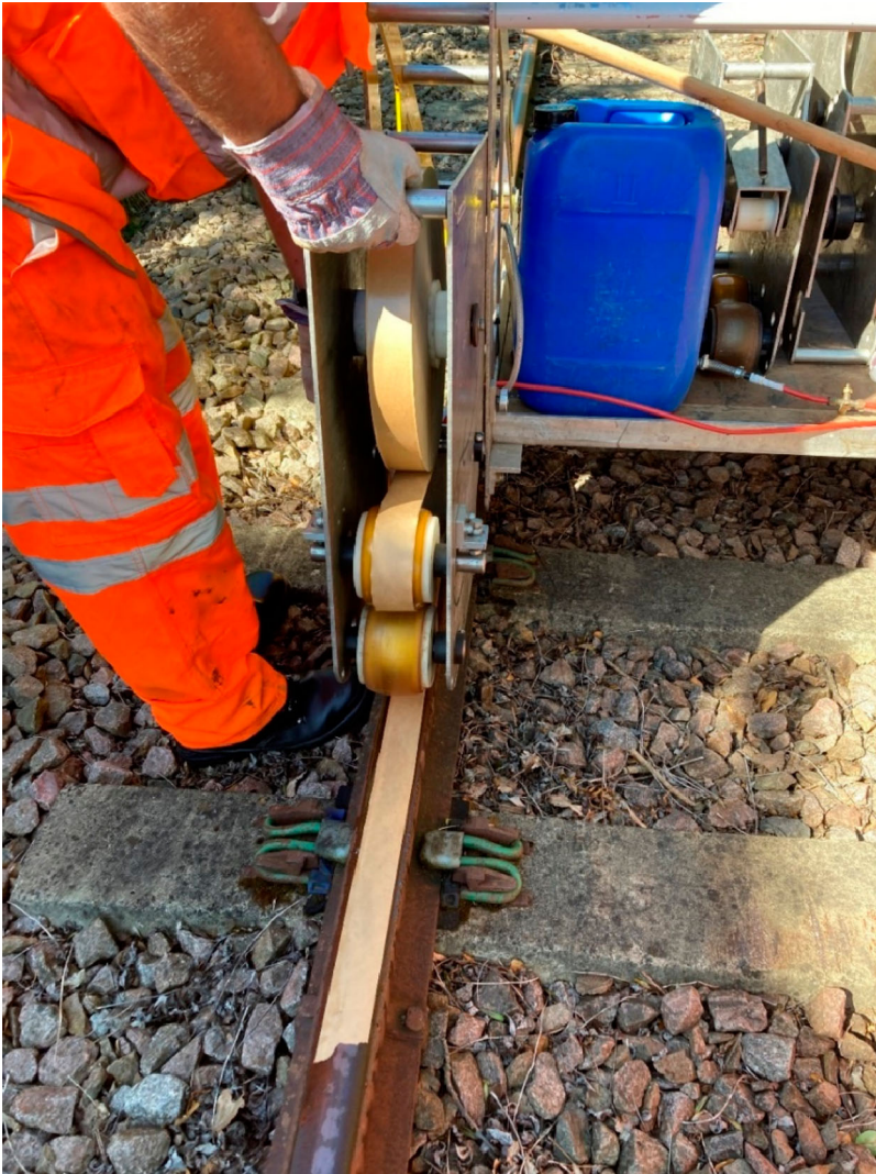
Figure 3. The tape laying trolley laying paper tape on the railhead.
