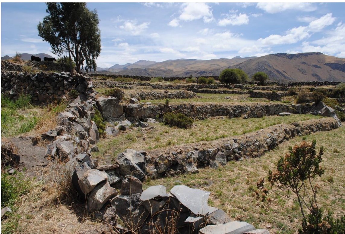
Figure 5.2 Rehabilitated terrace unit in Paccareta with external boundaries of larger dry-stacked volcanic rock and terrace faces of smaller stacked volcanic rocks topped with grassy berm, October 17, 2015 (photo by Alexander Menaker).
