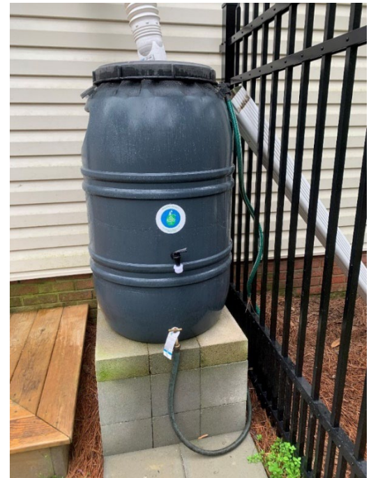
Rain Barrel Installed on Blocks
