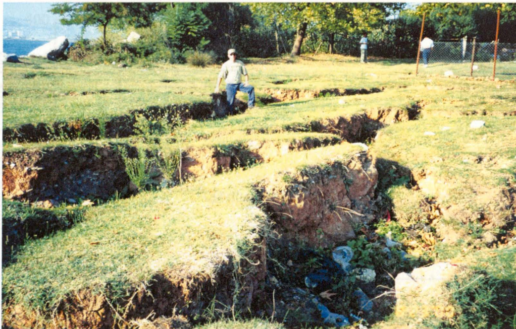
Figure 3.78 Photograph showing the large ground cracking that occurred at Police Station during the earthquake. The surface fault rupture exits the bay near here.
