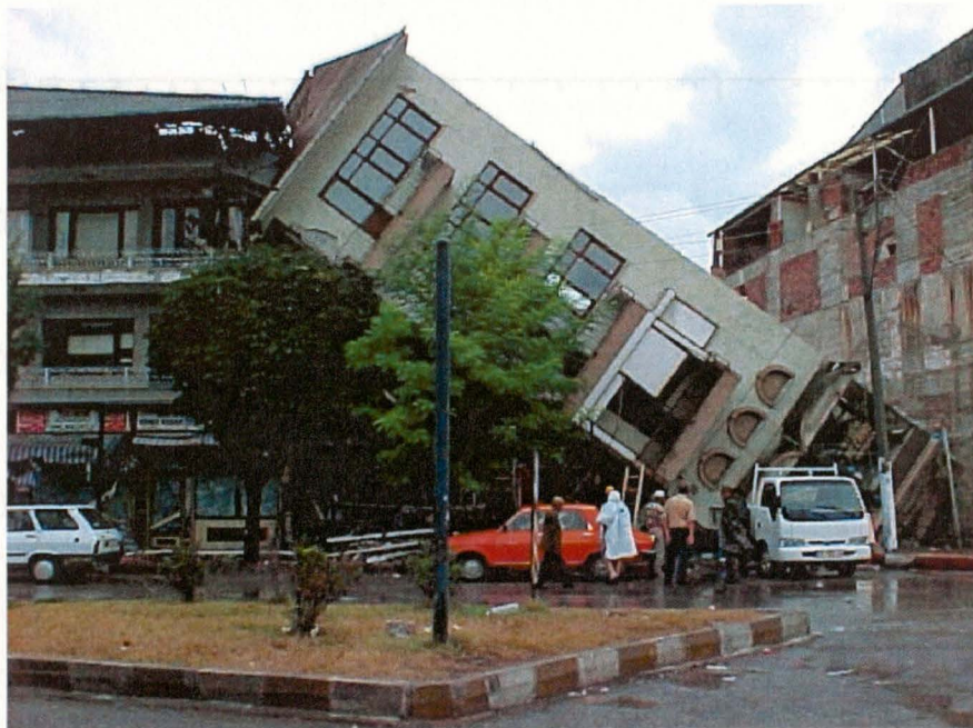
Figure 3.12 Photograph showing building B1 after it tipped over due to liquefaction of its foundation soil (from www.eerc.berkeley.edu/turkey/adapazari ).
