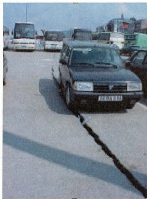
Figure 3.88 Photograph showing a lateral spread crack that developed in the paved parking area at Yalova Harbor. The cobblestone parking area was also damaged (from www.eerc.berkeley.edu/turkey/adapazari ).
