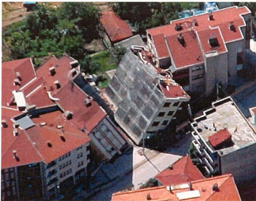
Figure 3.31 Photograph of Site G, where liquefaction of foundation soil caused buildings G2 (right) and G3 (left) to tip apart in a "V" (from www.eerc.berkeley.edu/turkey/adapazari ).
