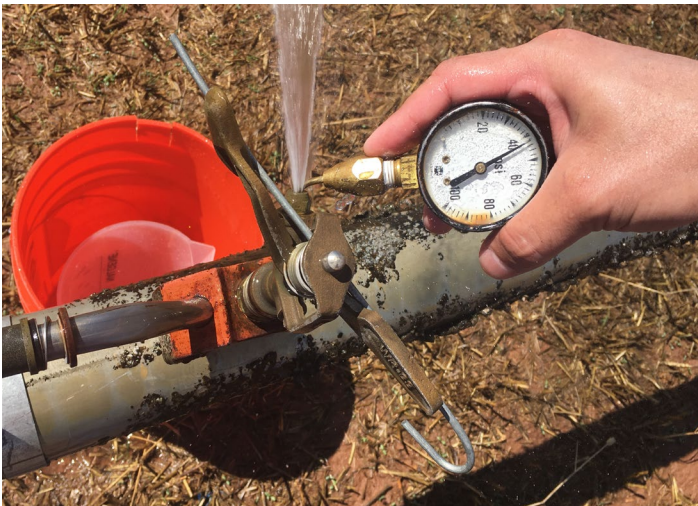
Figure 5. A Sprinkler Nozzle Pressure Reading Using a Pressure Gauge and Pitot Tube
