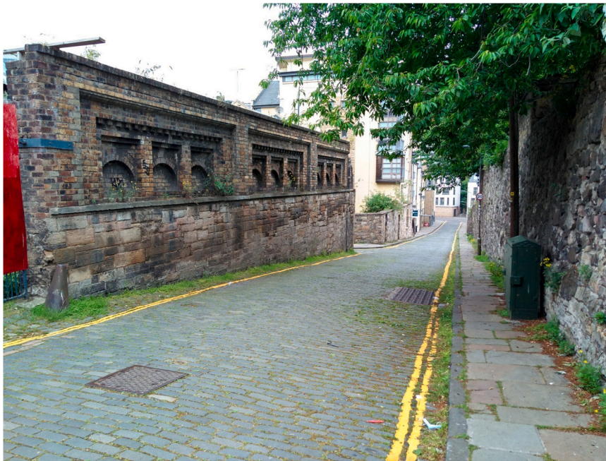
Fig. 4. The surviving eastern external wall of Gasworks on Tolbooth Wynd (left side), with blind openings (© Elizabeth Robson).
