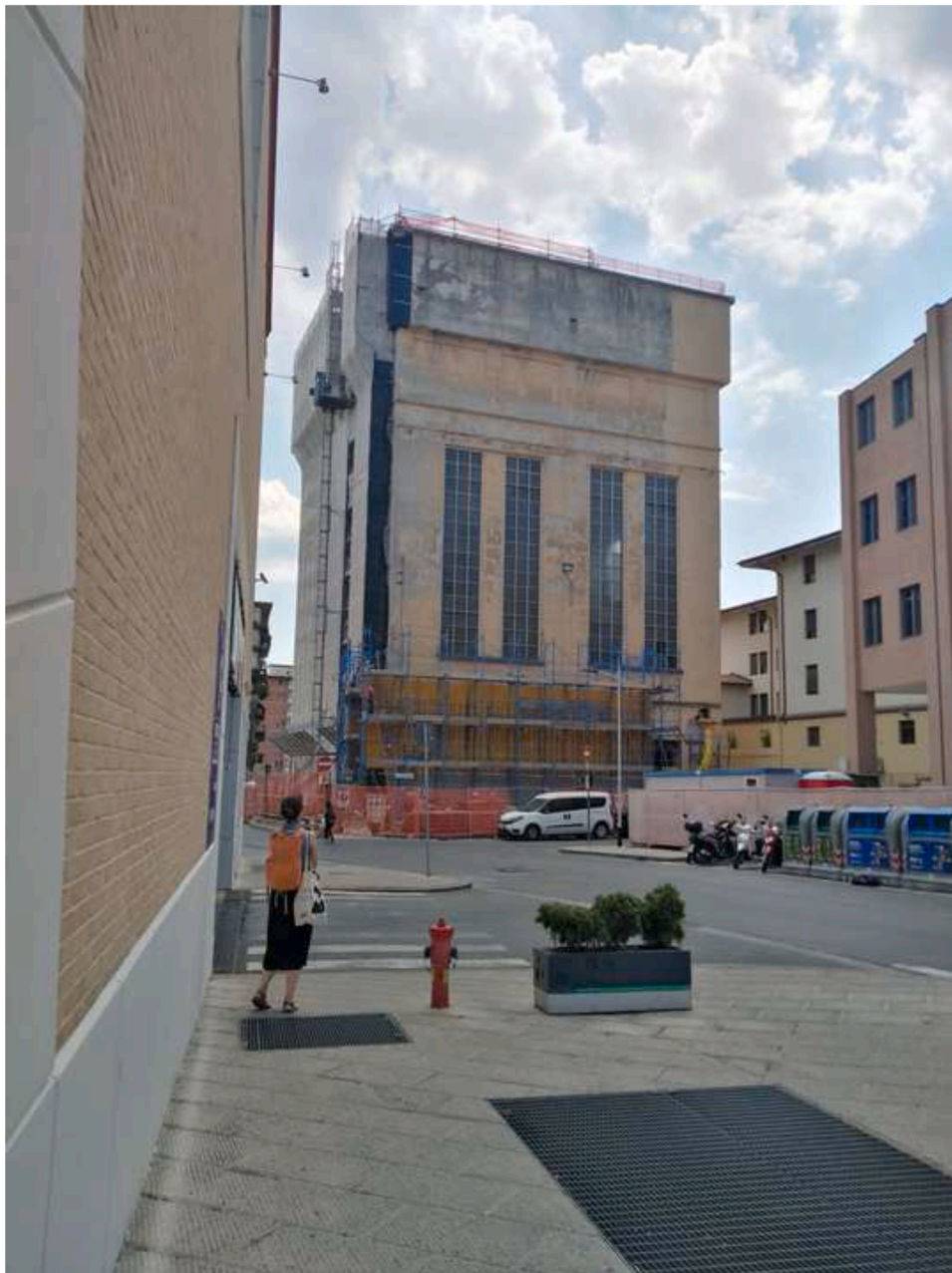
Fig. 22. The FIAT plant thermal tower (© Andrea Biondi).
