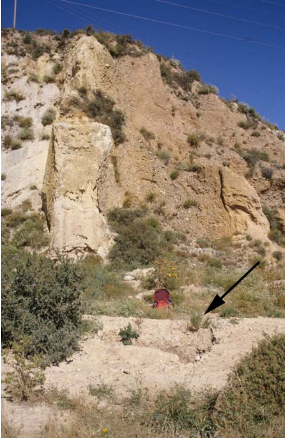
Figure 4. Collapse sinkhole developed next to a paleocollapse structure affecting Quaternary terrace deposits of the Alfambra River (Teruel Neogene Graben, NE Spain). This active sinkhole, affecting a recent artificial fill, most likely results from the reactivation of old cavities recorded by the adjacent paleosubsideance structures. Photograph taken on July 27, 1997.
