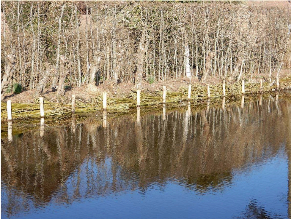
Figure 5: Willow branches for reinforcing the soft banks of a forest patch
