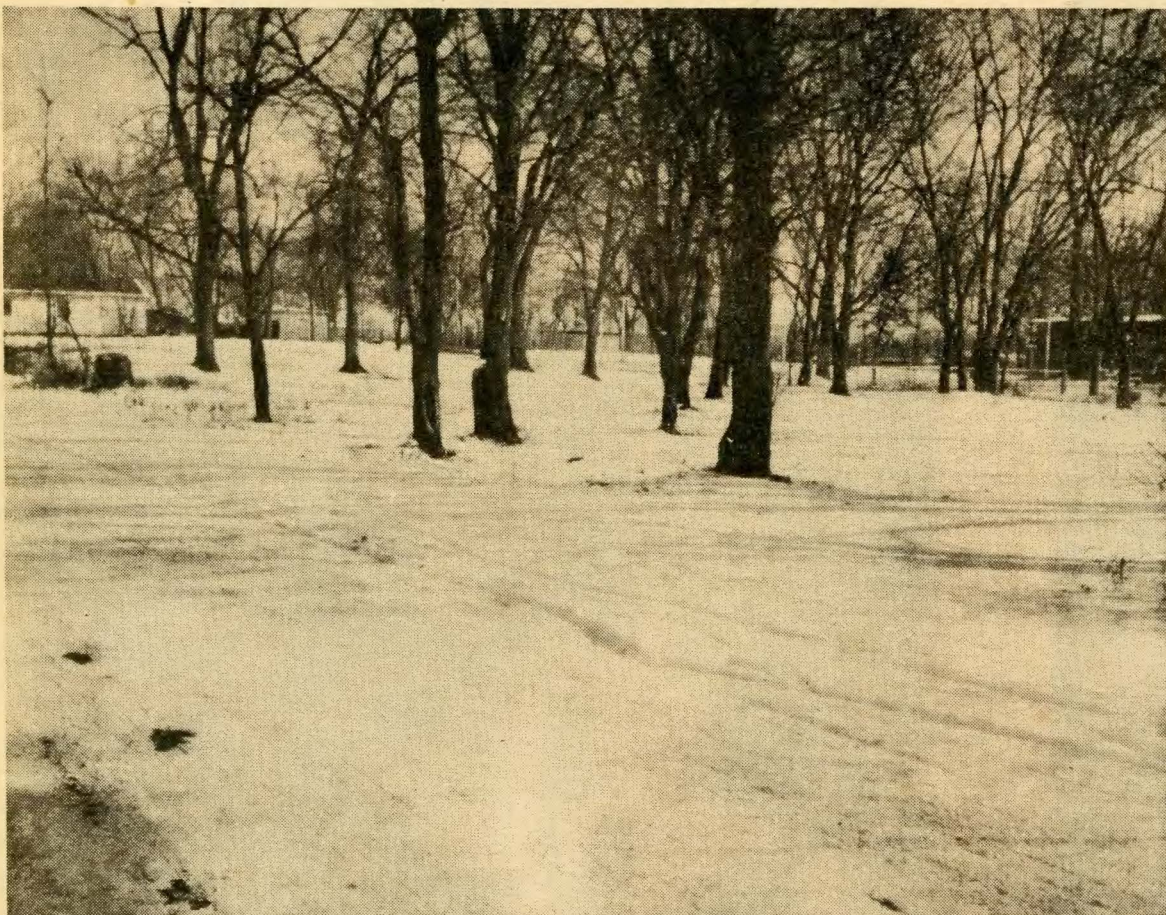
SNOW-COVERED vacant ground, which there is a lot of in the High Street area these days as work is nearing completion on the removal of all sub-standard housing in the Parkside East project. Only a few homes remain to be torn down according to officials of the Urban Renewal office.
