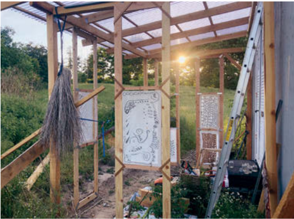
Fig. 6 The Tiny House with its extension in which the textile hybrids are set up as facade elements.
