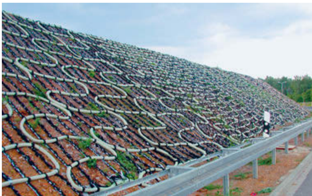
Fig. 3 ↑ Geotextiles using Kemafil® coarse rope structures as reinforcement for landscaping to prevent erosion in road banks.
