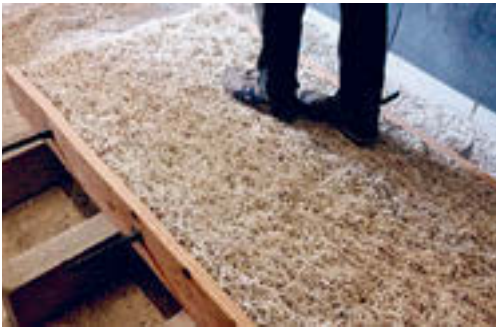
↑ The wall-slab was formed by fabricating a vertical superjammed wall, rotating into the horizontal.
