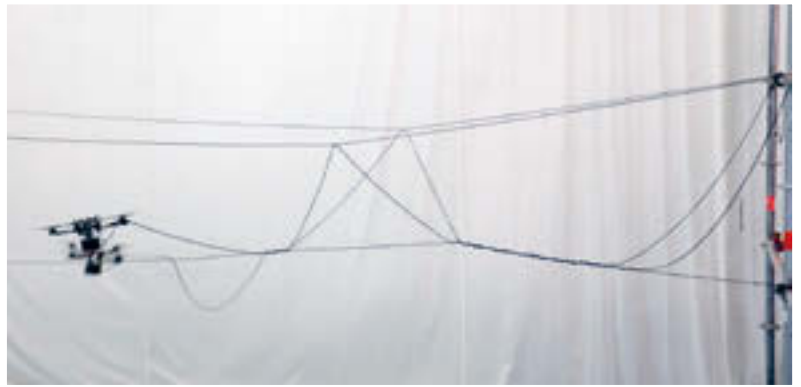
↑ Simultaneous erection of the three main links by three vehicles. Two machines start building the handrails on one side, while the third machine fixes the footrope on the other.
