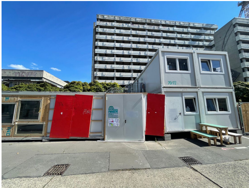
Fig. 4. The façade of Razam headquarters in a temporary make-shift squat during the reconstruction of the Haus der Statistik. View from Otto-Braun-Straße.
