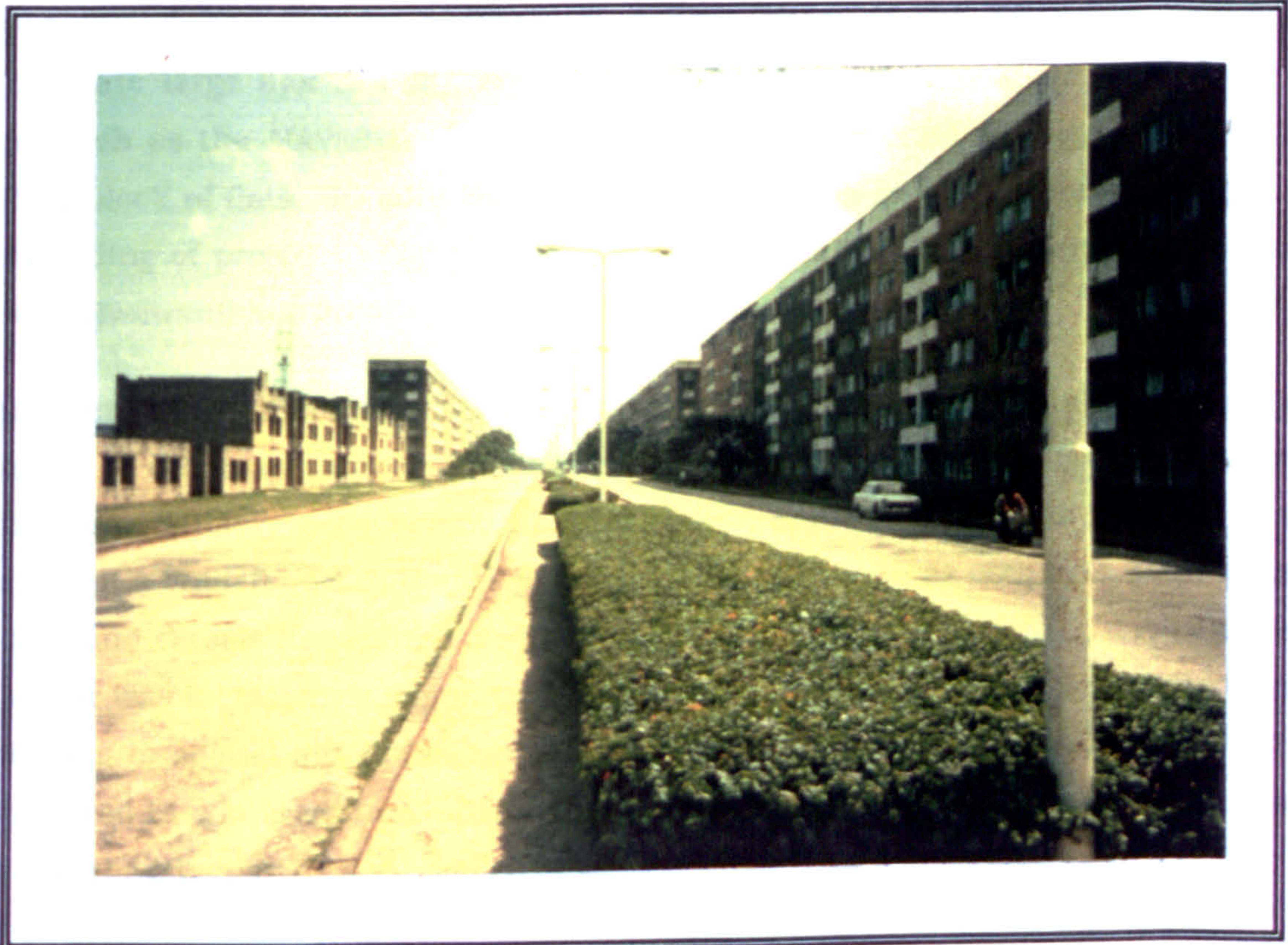
Plate 6 Michenzani Housing Scheme with empty dual carriageway
