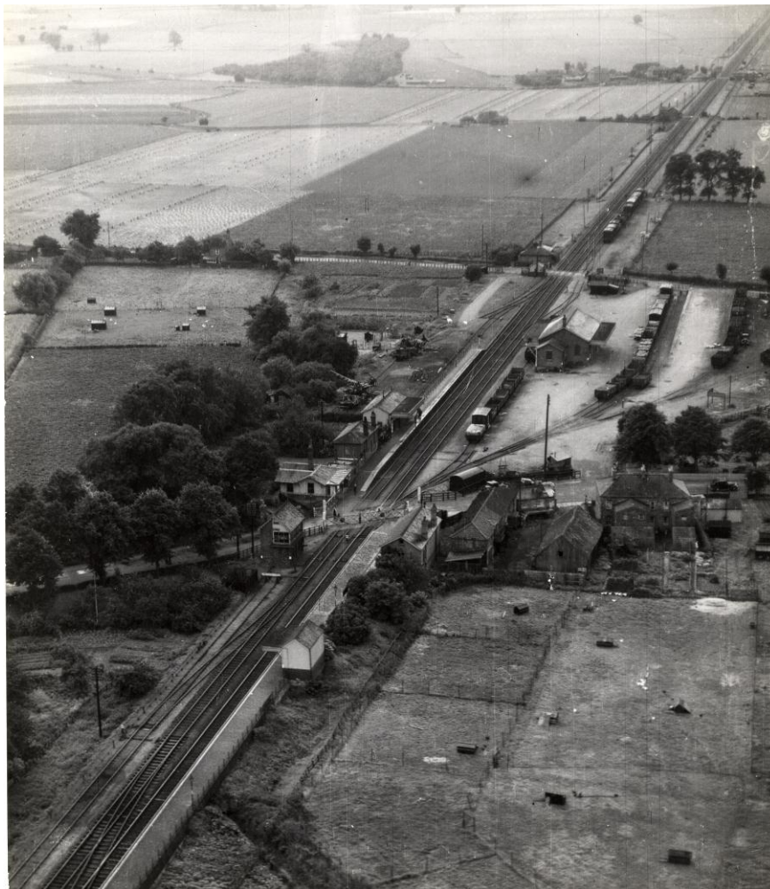
Figure 25. Aerial view of railway gun experiment - H.B. Cott
