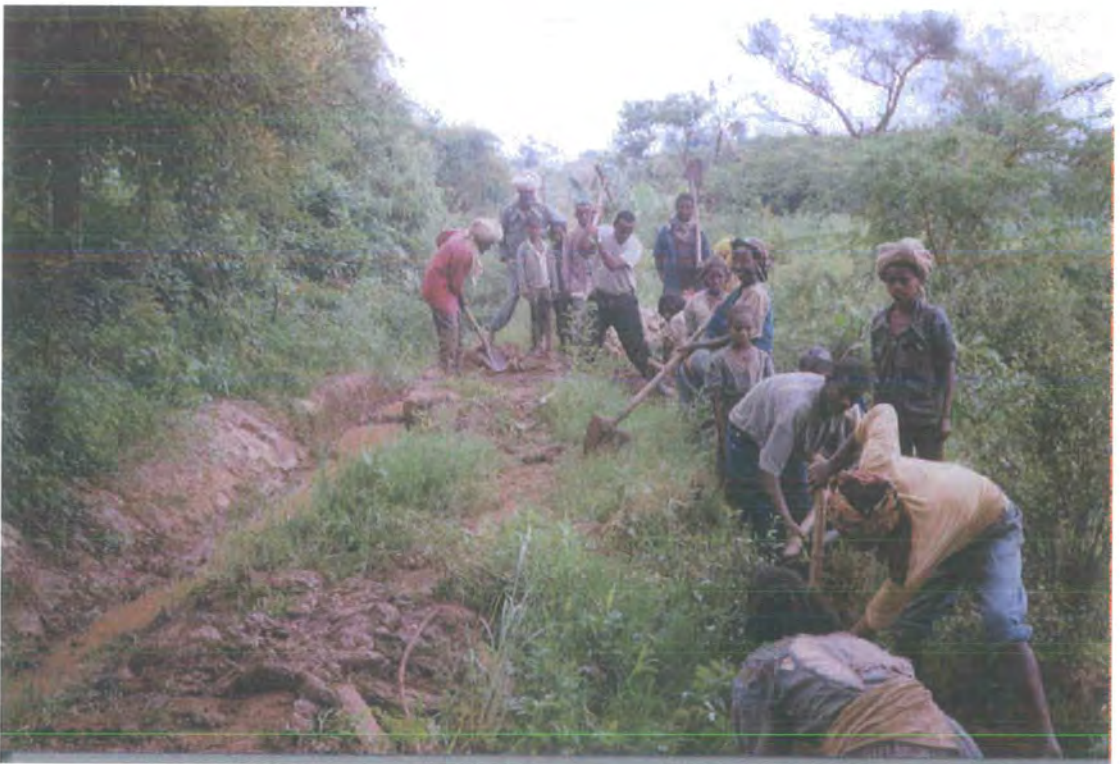
Plate 6.1. Digging a drainage canal (below) and a crossing canal (above) to cultivate more land on the other side of the gully below the dam.
