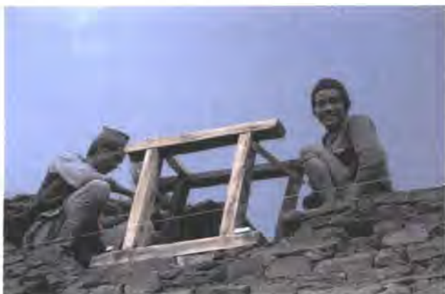
Plate 4.4: Men constructing a house in Turana in Phagun
