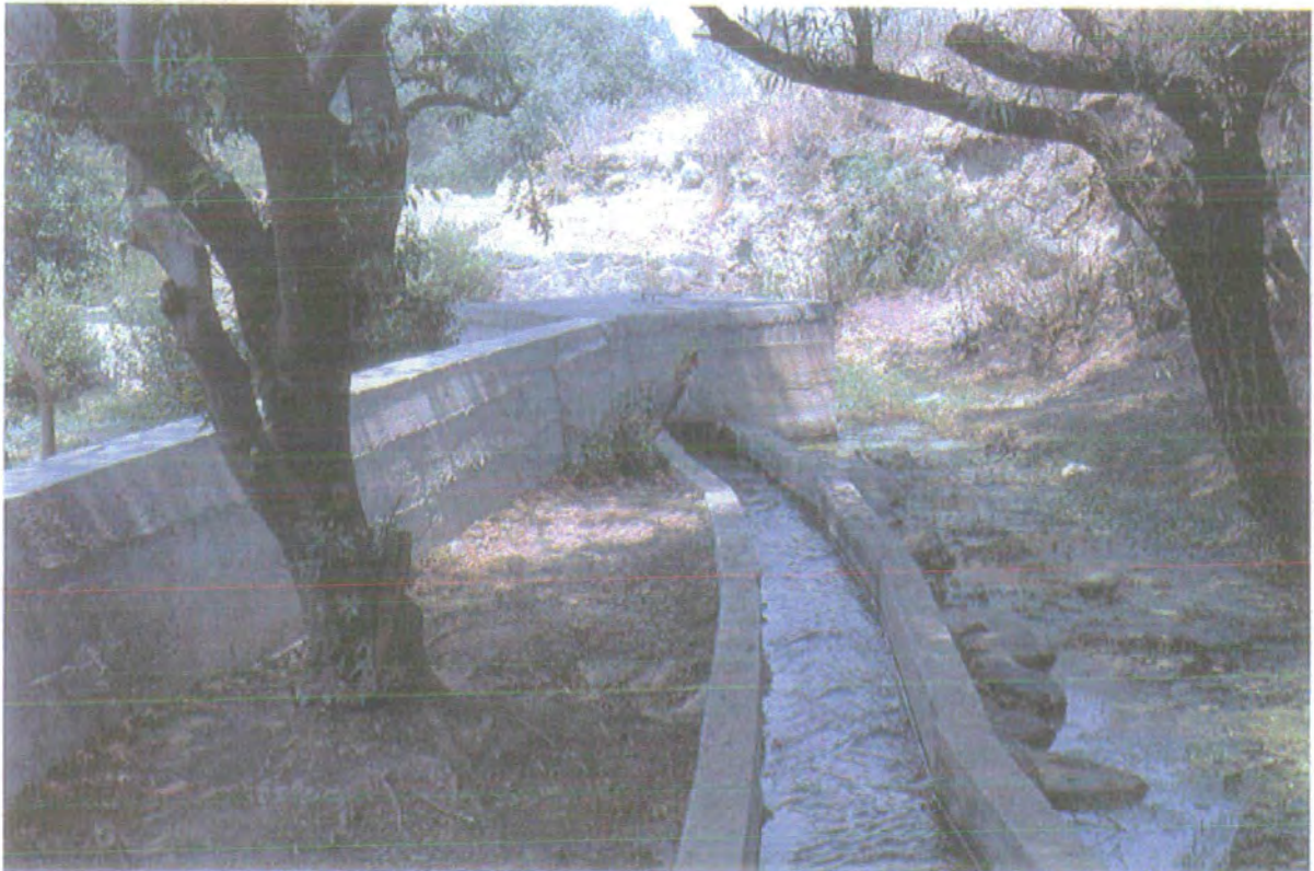
Plate 6.8 Infrastructure for irrigation in the ejido of Santa Maria Nativitas, (programme Alianza para el Campo, 1997)
