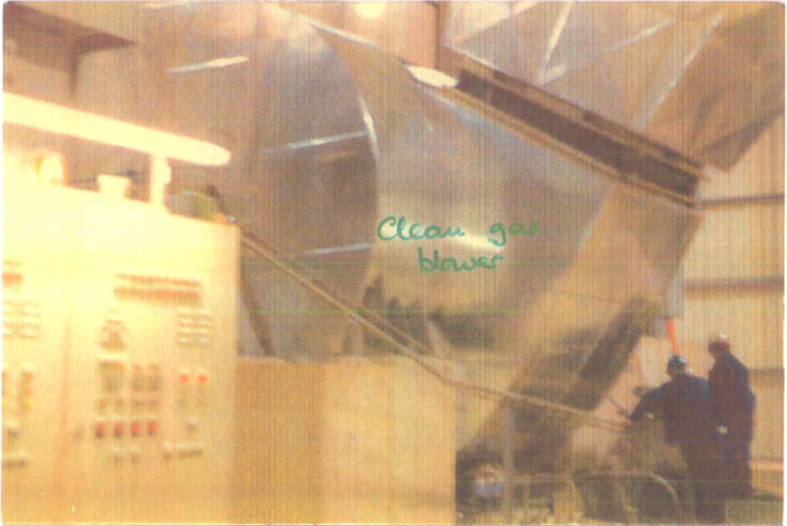
Illustration 7 Clean flue gas blower
