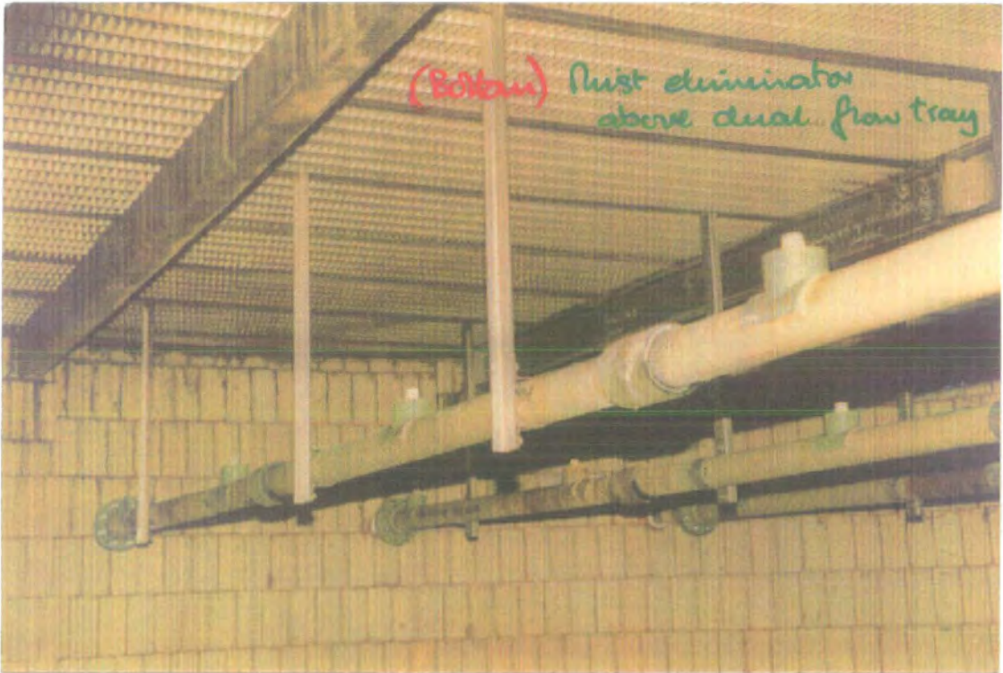
Illustration 5 Mist eliminator downstream of dual flow tray
