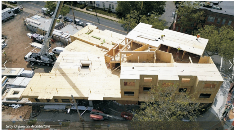
Fig. 4. 340+ Dixwell, View from construction site, Source: https://www.woodworksinnovationnetwork.org/en-ca/projects/340-dixwell-ave
