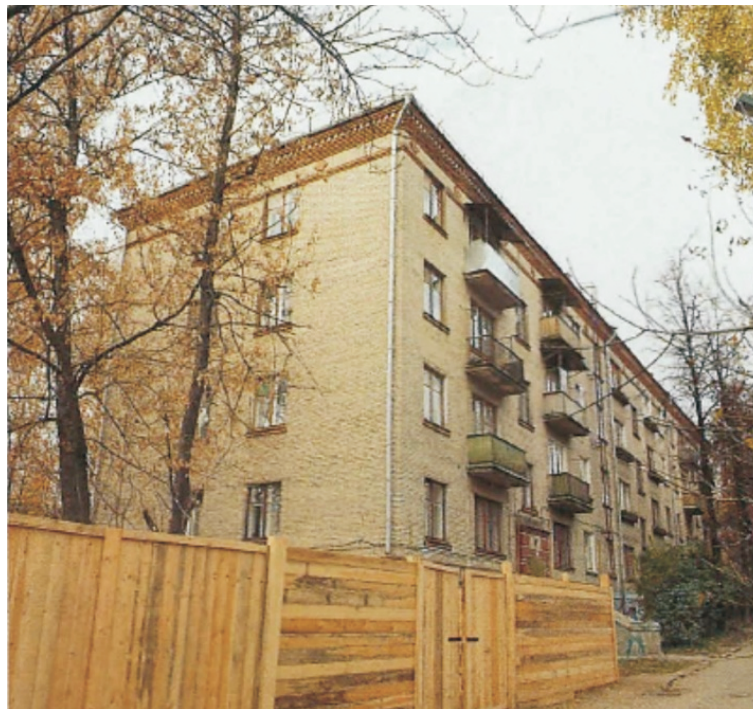
Fig. 6. The existing building before reconstruction, Source [7]
