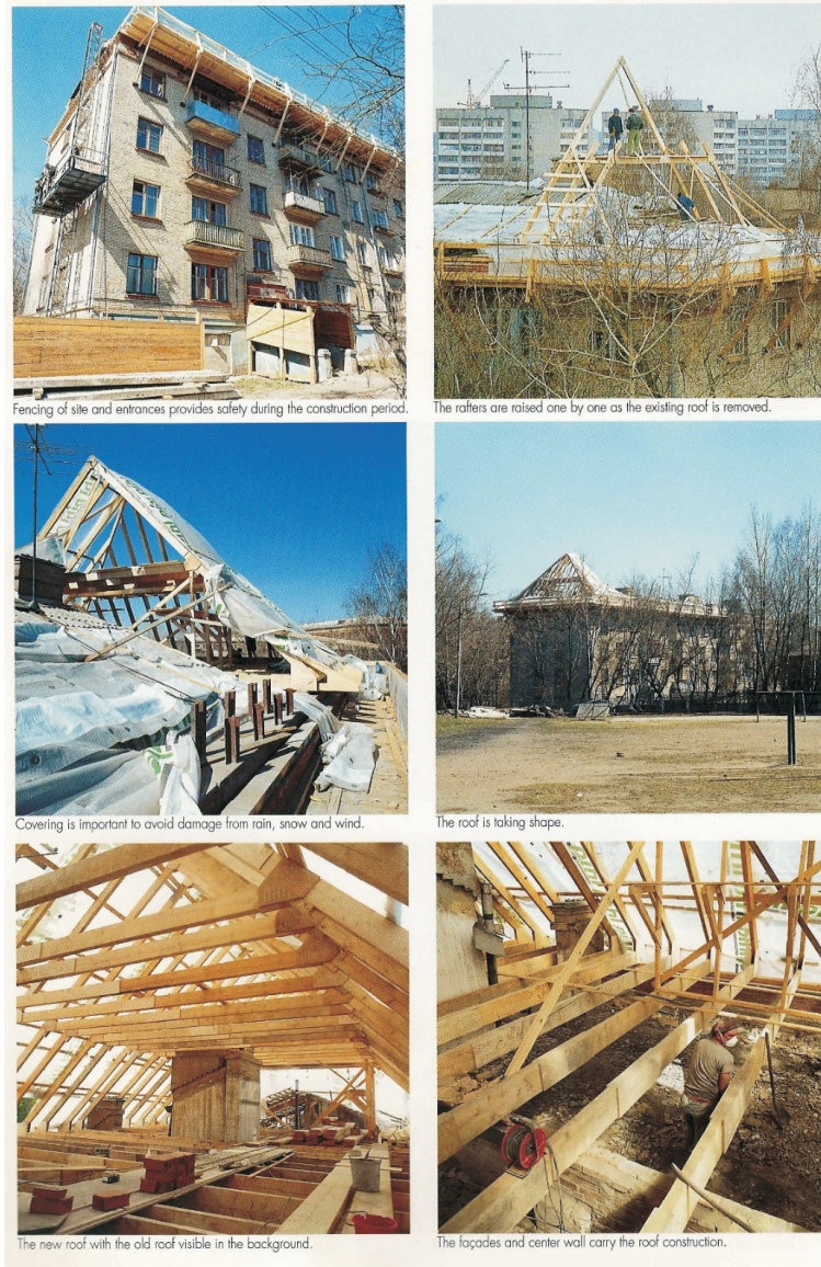
Fig. 10. Pictures from the construction stage, Source [7]
