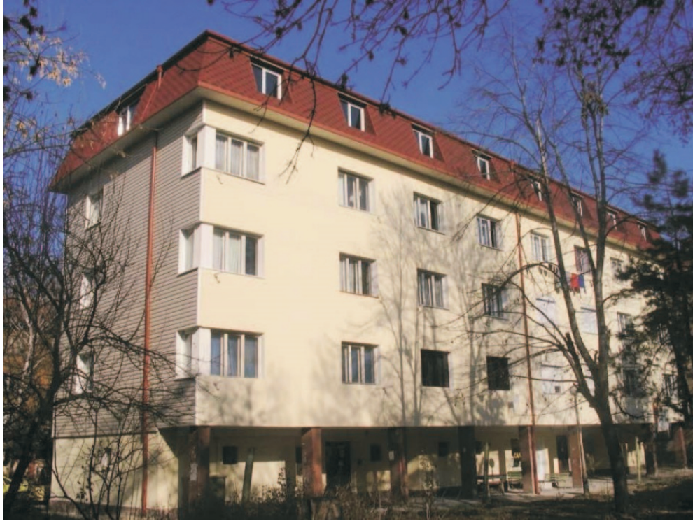
Fig. 13. Completed pilot building in Zaharna Fabrika , Source [11]
