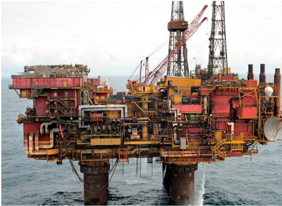
Figure 1.2: A typical offshore platform
