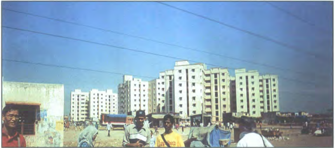
Figure 20: New Slum Rehabilitation Authority (SRA) buildings in Mankhurd, Mumbai, November 2002
