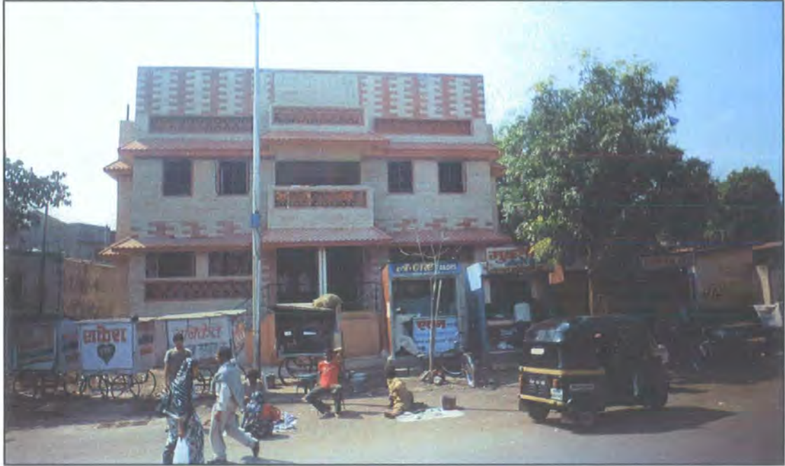
Figure 16: 'Prasadsan Palace' toilet block, Pune, November 2002.
